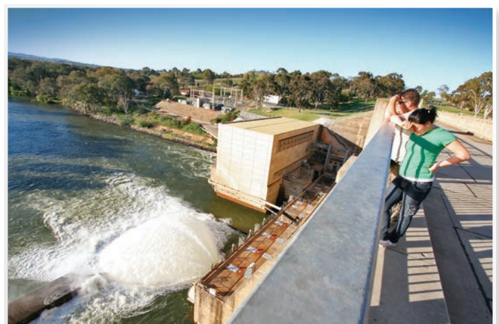
The powerful spill at the Hume Reservoir
